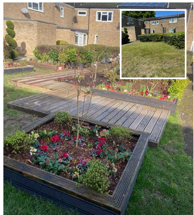
Coventry Close after works (inset: before)
