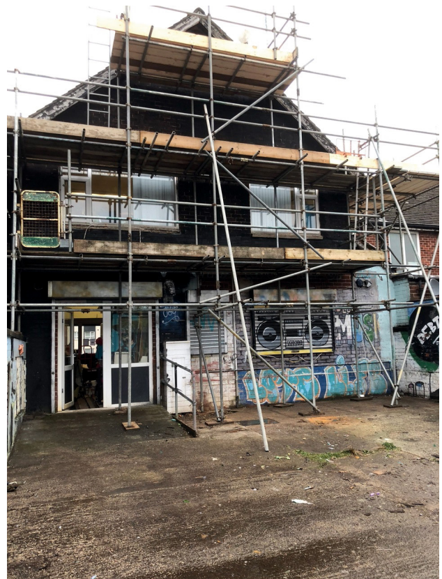
Retrofit works beginning at Soundskills April 2024
