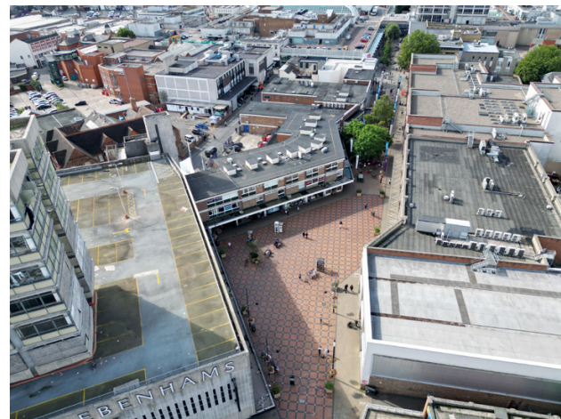
Swindon Town Centre Rooves by Drone
