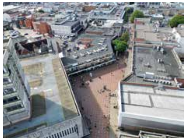
Swindon Town Centre Rooves by Drone
