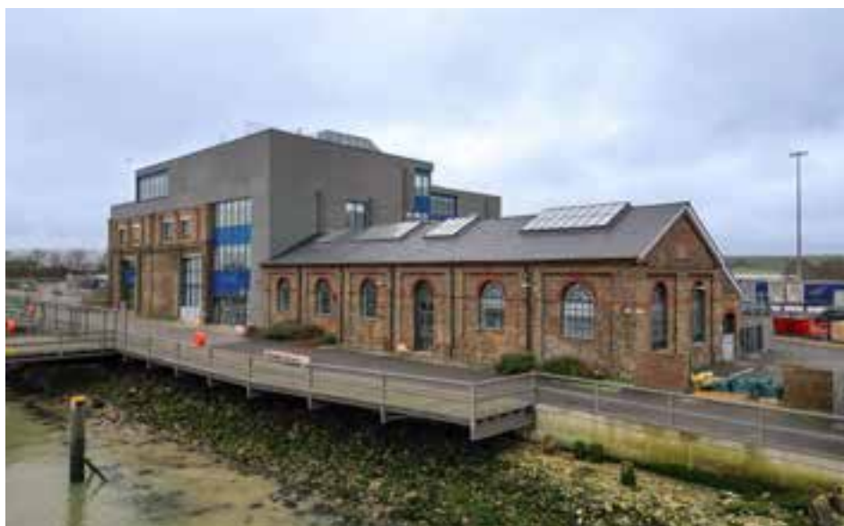
Marine Workshops, former technical college and new site of council offices in Newhaven
