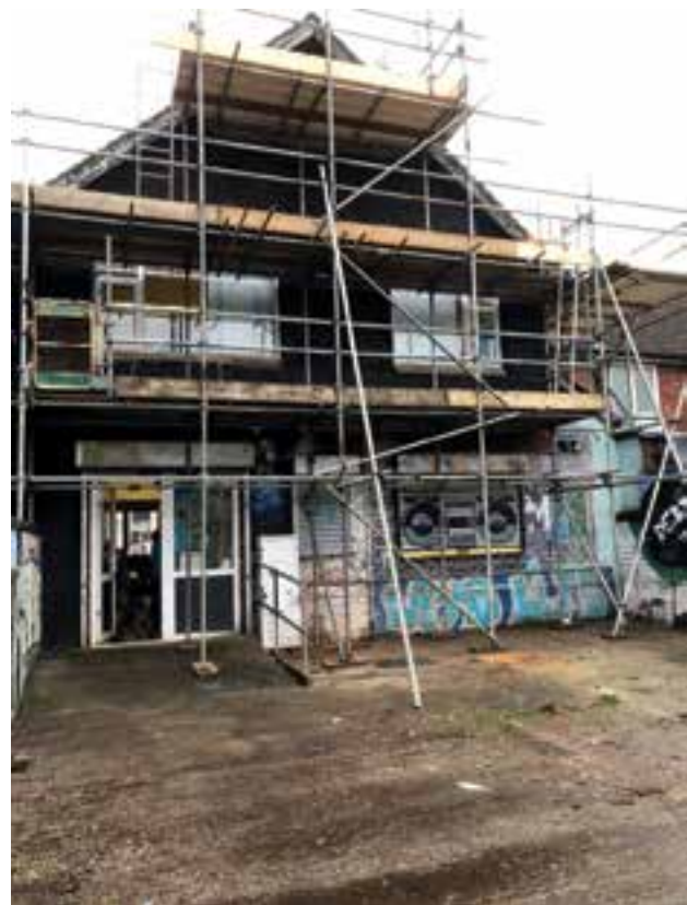
Retrofit works beginning at Soundskills April 2024
